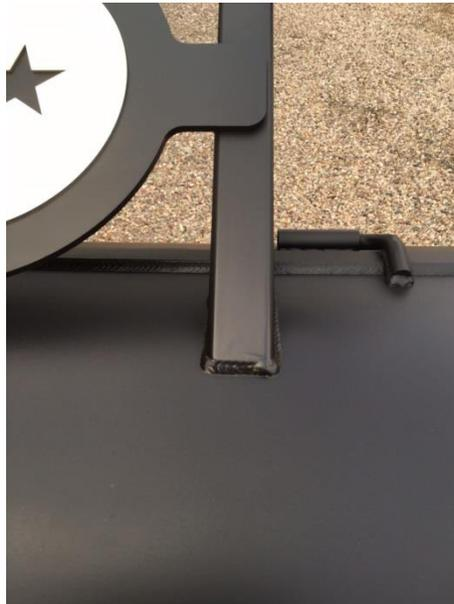
The second example of paint repair, is not actually paint damage, but rather a surface defect in the metal under the paint. The following pictures illustrate the defect prior to repair.
